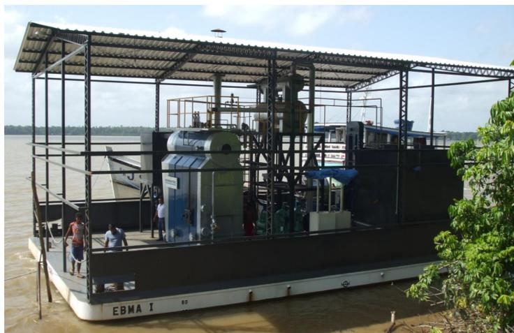
*Figure 19: Mobile biomass power unit based on Rankine cycle (50 kW) in the Amazon region. Source: (Nogueira, 2012)*
