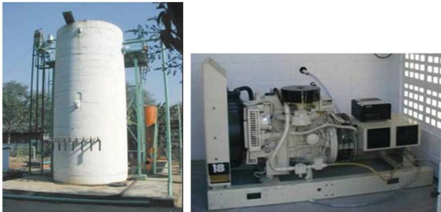
*Figure 32: UASB Biodigester and Engine Cycle Otto of 18 kW. Source: (Pecora, 2006)*
