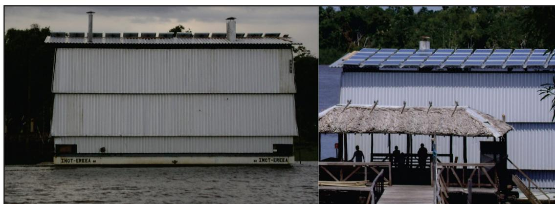
Figure 20: Mobile power unit project hybridized with PV panels. Source: (Nogueira, 2012)
