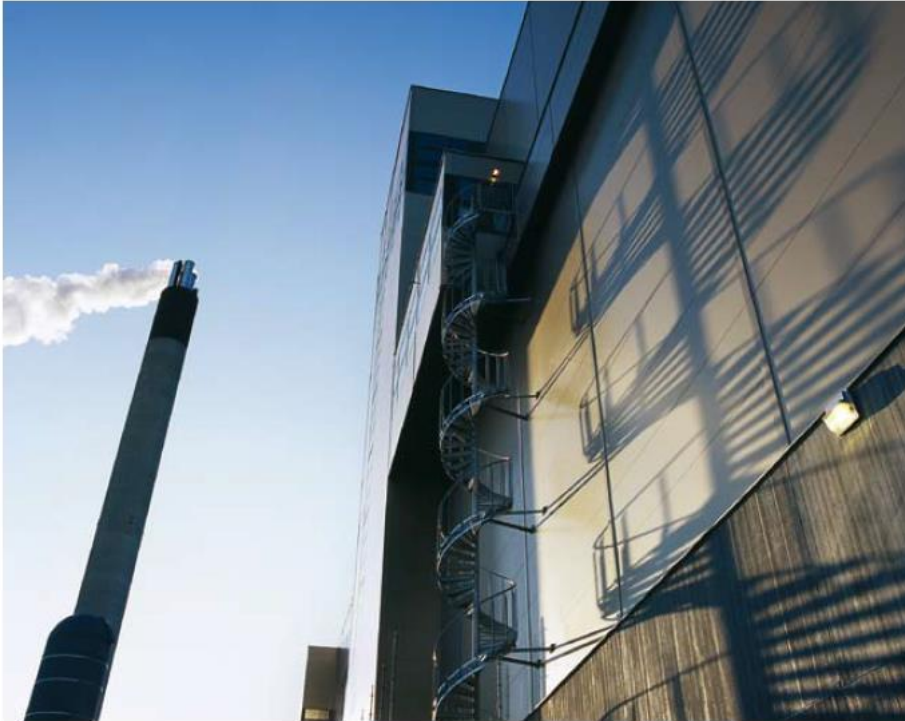
In 2006, the combined heat and power (CHP) plant for waste fuel at Korsstaverket in Sundsvall became operational. Photo: Torbjörn Bergkvist
