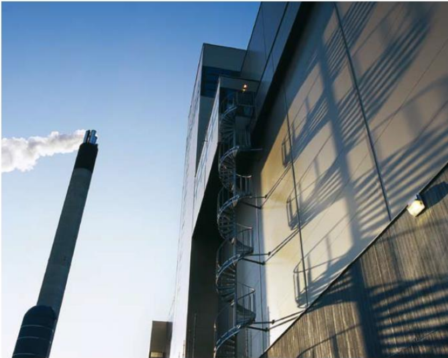
In 2006, the combined heat and power (CHP) plant for waste fuel at Korsstaverket in Sundsvall became operational. Photo: Torbjörn Bergkvist
