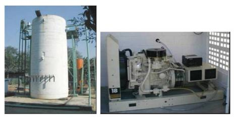
Figure 32: UASB Biodigester and Engine Cycle Otto of 18 kW. Source: (Pecora, 2006)
