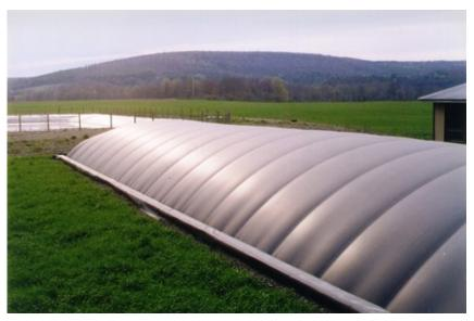
Figure 34: Photo of Biodigester Covered Lagoon<sup>34</sup>
