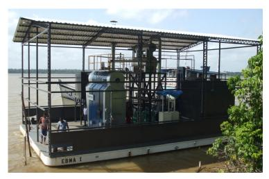
Figure 19: Mobile biomass power unit based on Rankine cycle (50 kWe) in the Amazon region. Source: (Nogueira, 2012)
